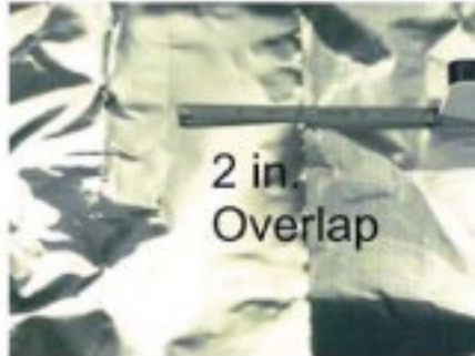
Overlap the two pieces by 2" – lengthwise.
