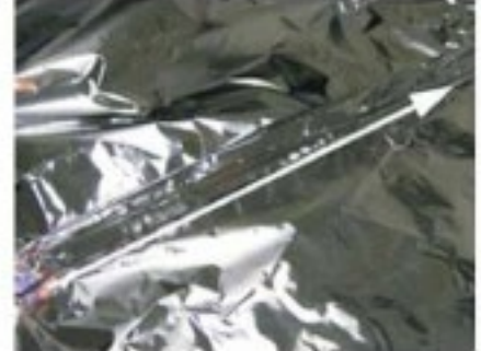
Lift the overlap, crease and fold flat for the length of the seam (26").
